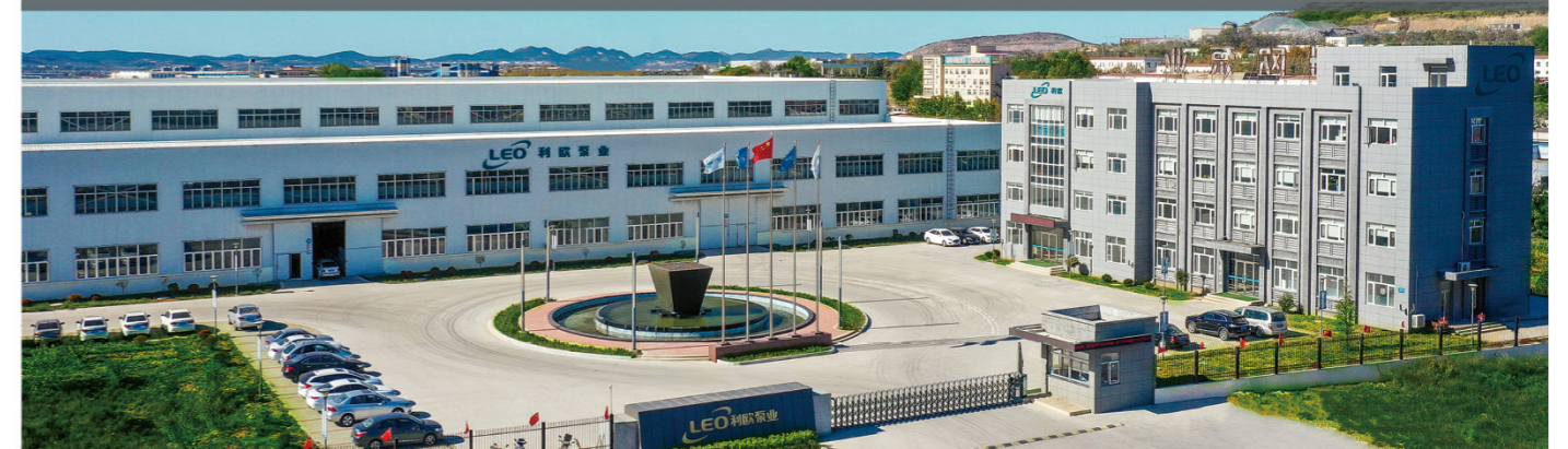
Pump Manufacturing Base for Petrochemical Industry
